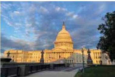
Washington DC ARX USA, Inc. 609 H Street NE, Suite 433 Washington DC, 20002 US
